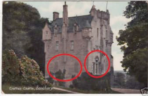
[PC 0001] Crathes Castle c1908 West facing windows are filled in and south facing windows are altered to have squared off tops.
