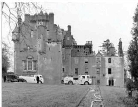
[PH 0017] Crathes Castle 1966 Fire destroys Victorian wing.
