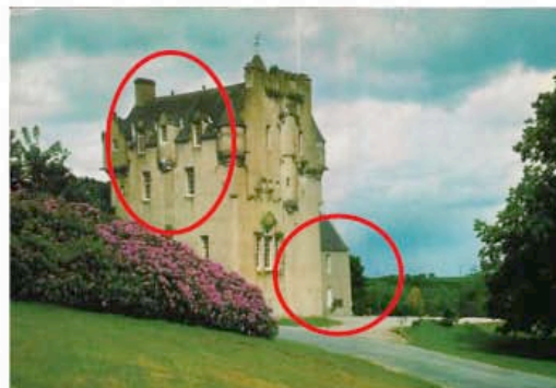
[PC 0026] Crathes Castle 1975 After the fire the NTS add a new east replacement wing which returns it to the original two story model. Chimney removed to West wall of tower
